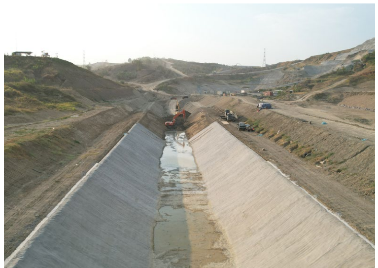
Anchor trenches backfilled with non-erodible fill
