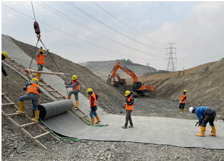
CCX-M® laid transverse across the channel
