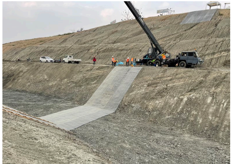
Crane used to deploy CCX-M® transversely
