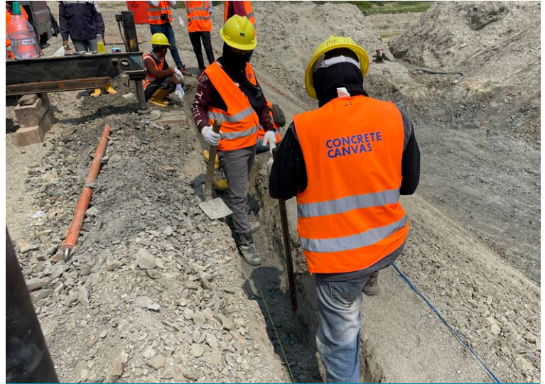
Anchor trenches dug at the shoulder of the channel
