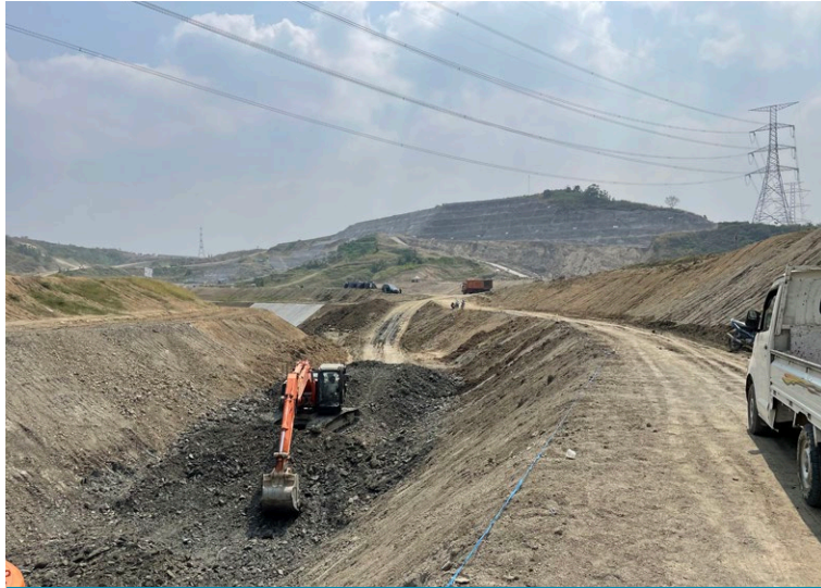
Channel excavated to specification
