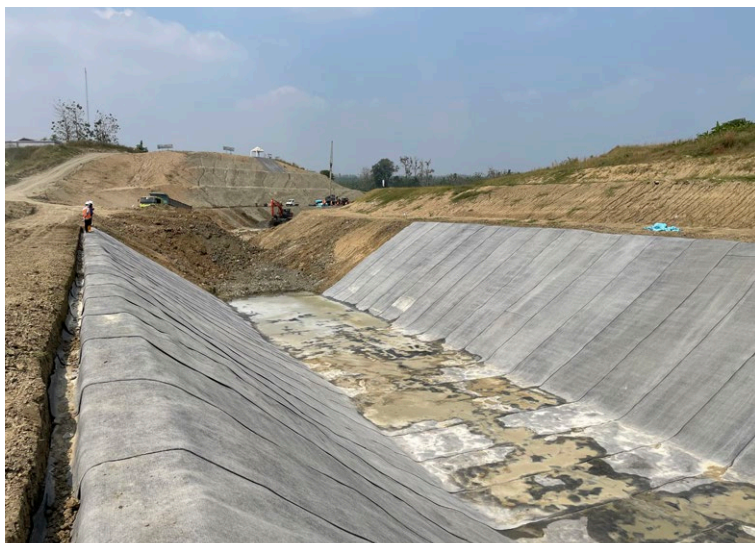
CCX-M® secured within anchor trenches
