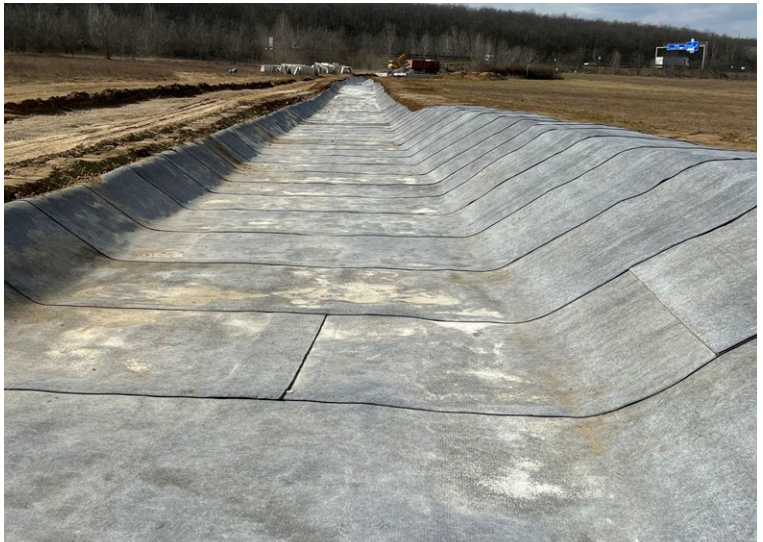
Completed section of channel including the use of CCX-M™ offcuts
