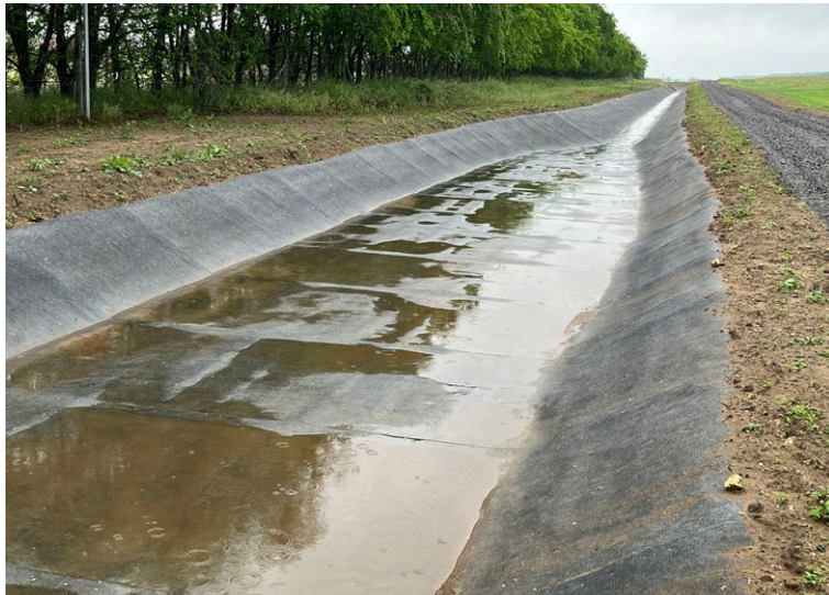
Section of channel showing profile change
