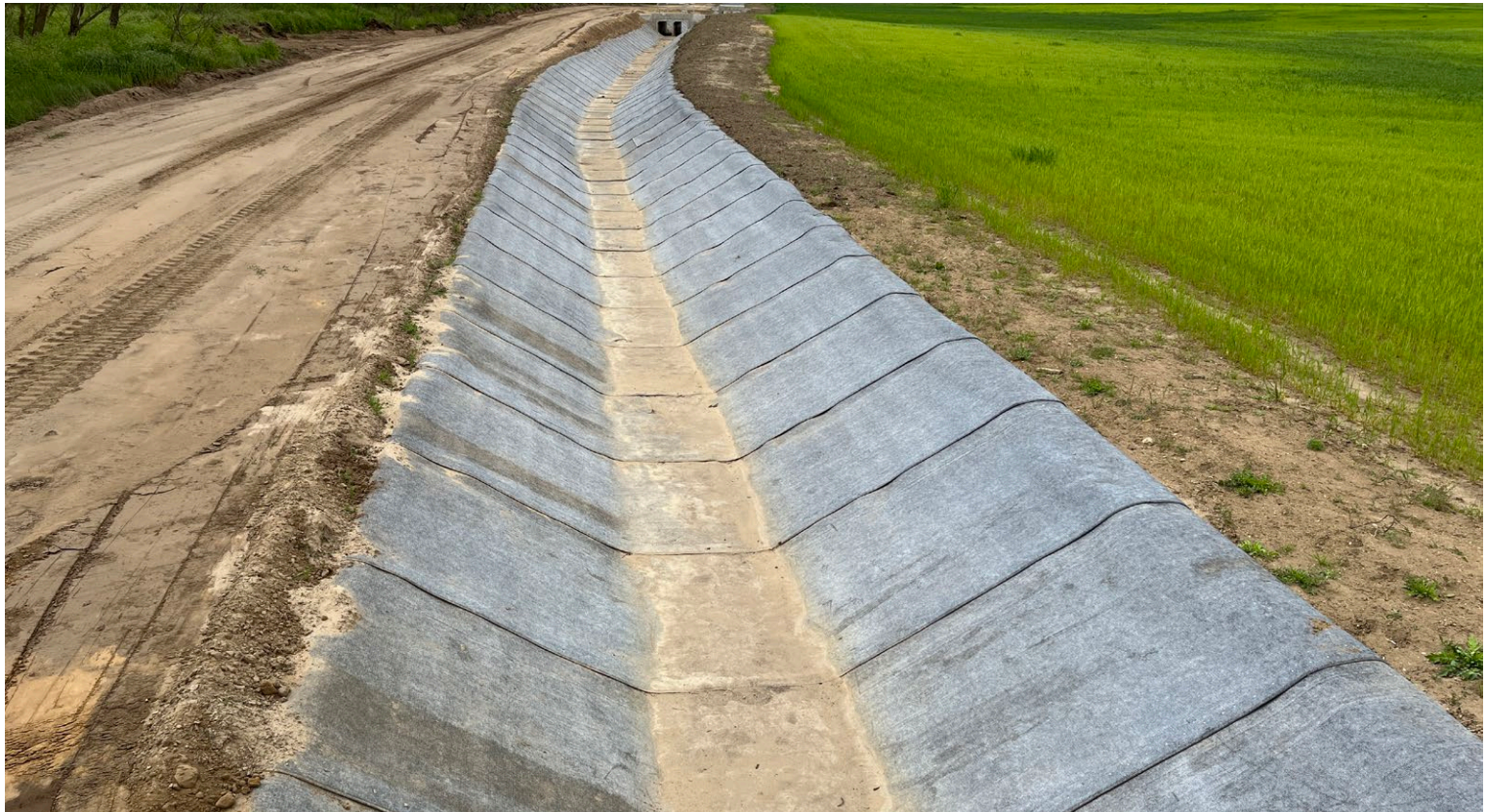
Completed section of channel
