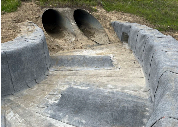
Baffles and gabions lined with CCX-M™
