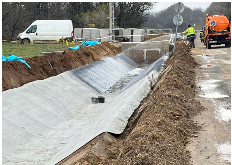
CCX-M™ hydrated using a water bowser and hose
