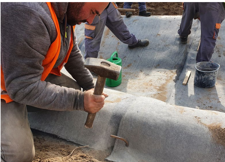
CCX-M™ secured with J-pegs within anchor trenches
