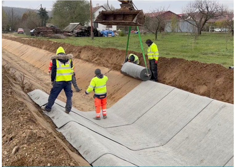
CCX-M™ laid transversely across the channel
