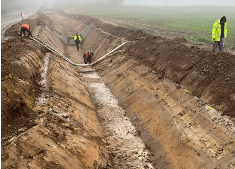
New profile cut to specification
