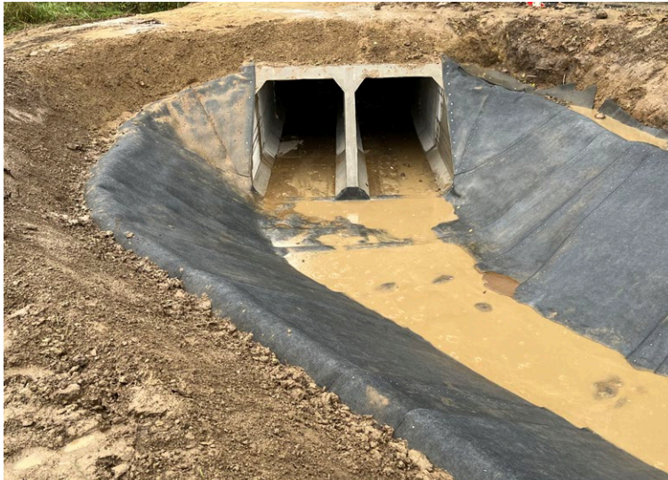
CCX-M™ terminated onto culvert headwall
