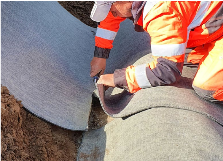
CCX-M™ cut to length using hand tools
