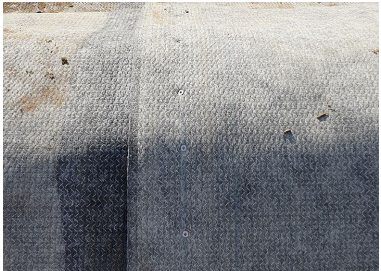
Layers of CCX-M™ overlapped and secured using screws 100mm apart
