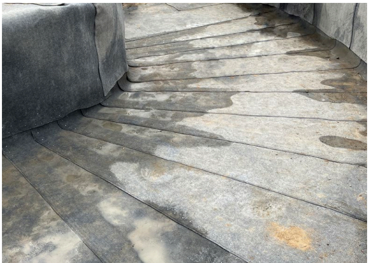
Completed 90° bend section with pie pieces
