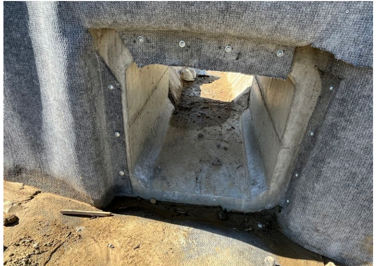
CCX-M™ terminated onto culvert headwall
