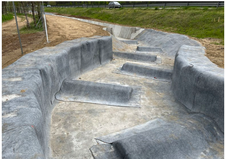
Baffles and gabions covered in CCX-M™
