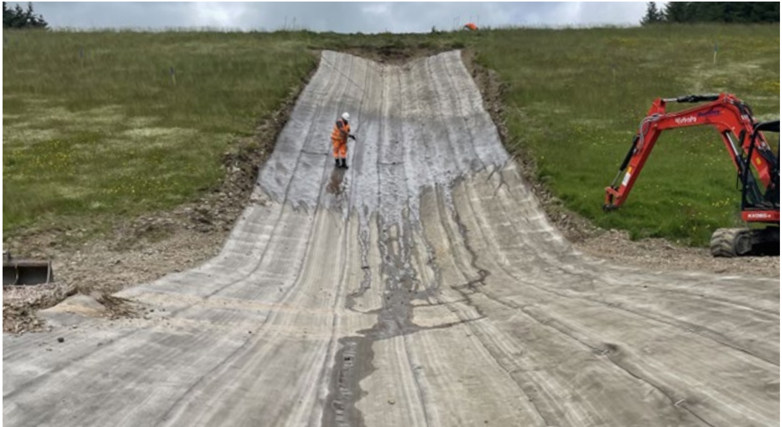
CCT1® being hydrated using water from the reservoir
